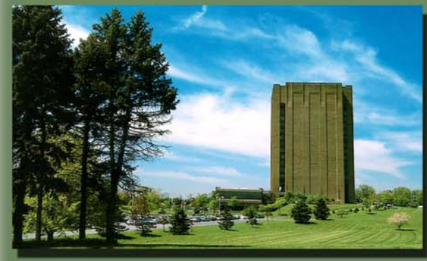
National Agriculture Library Abraham Lincoln Building, Beltsville, Maryland
